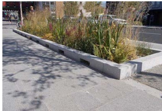
Sustainable urban drainage diverting surface water runoff to support urban greening.
