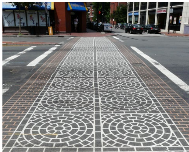
Options for artistic intersections when entering East Street could be explored using thermoplastic paint and stencils.
