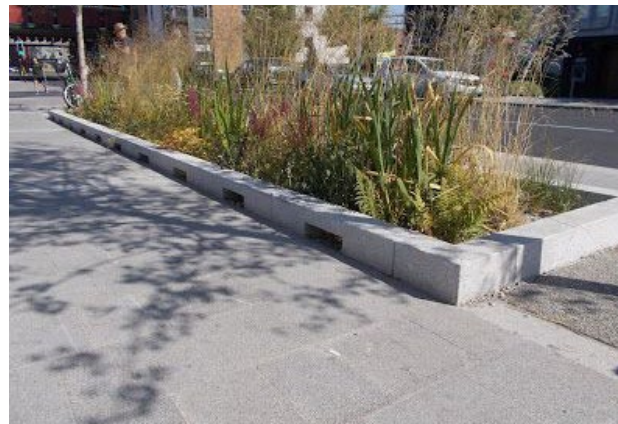
Sustainable urban drainage diverting surface water runoff to support urban greening
